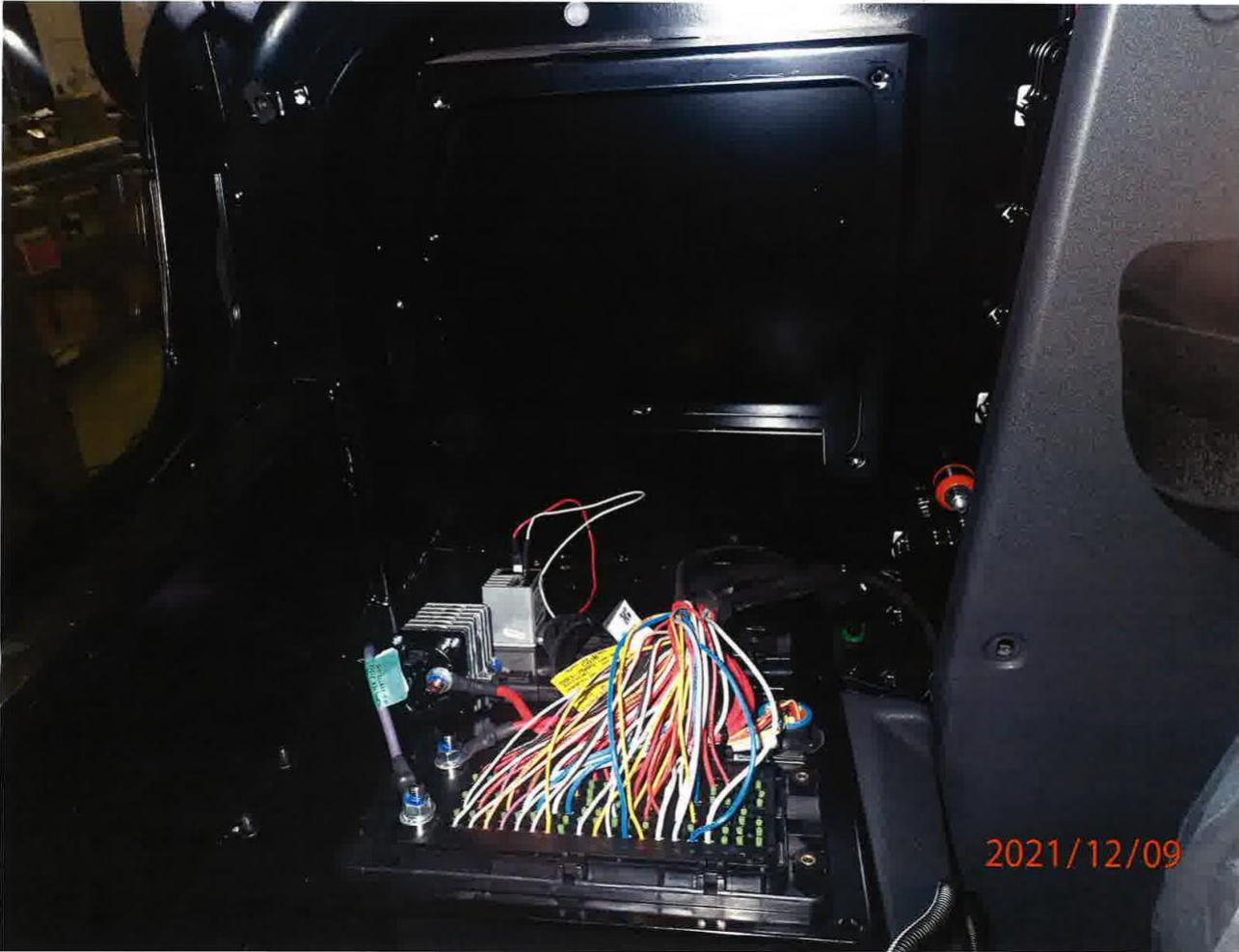
iv. Fuse panel back
